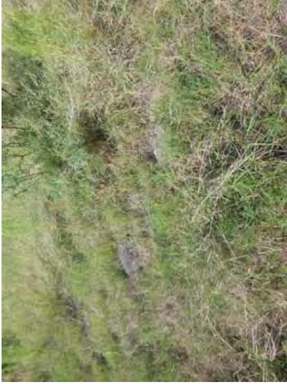
Photo 94: Loose soils on east embankment exterior slope.
