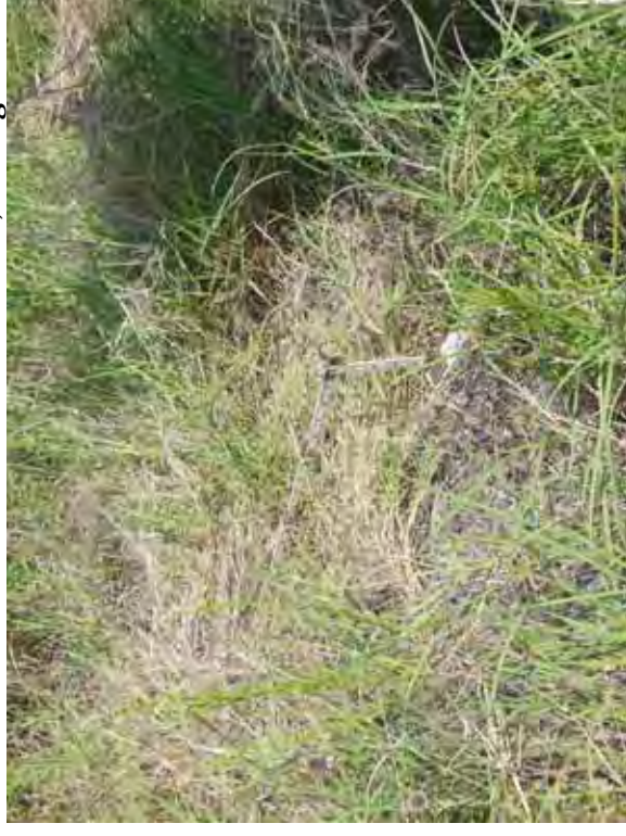
Photo 97: East embankment exterior slope measured approximately 4H:1V.
