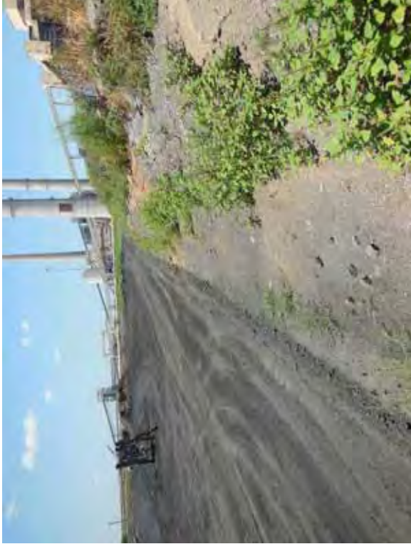
Photo 26: NP/SP - Erosion of ash material on common embankment south slope, looking west.
