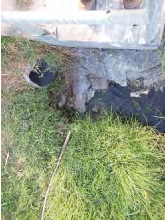
Photo 89: SP – 12-inch-diameter piping at outfall 103B.
