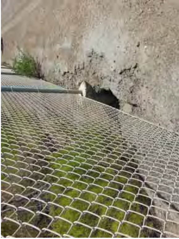
Photo 5: NP - North embankment exterior slope, looking northeast. Note erosion near fence post.
