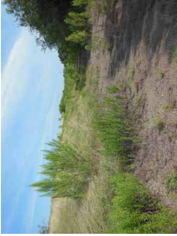
Photo 95: East embankment exterior toe, looking north.
