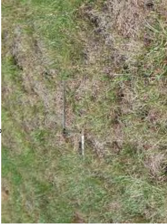
Photo 63: SP – Approximately 3H:1V side slope at south embankment exterior slope.
