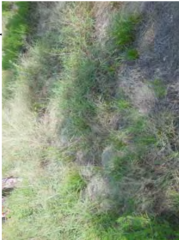
Photo 96: Loose soils near east embankment exterior toe.
