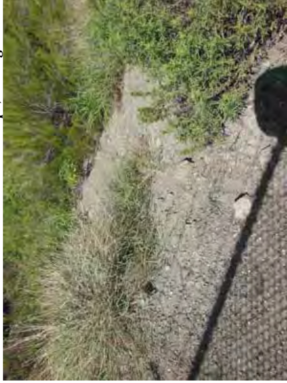
Photo 51: NP - Erosion on north embankment exterior slope, looking north.
