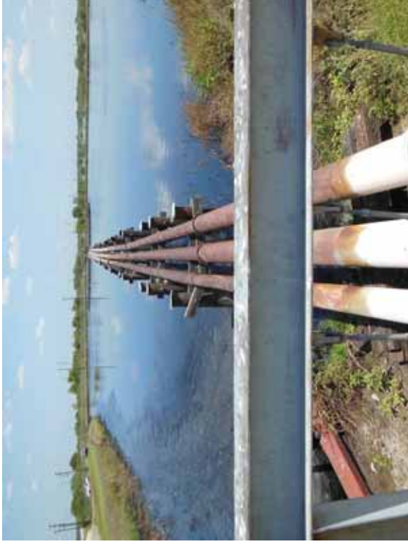
Photo 33: NP - Inlet pipes at southwest corner. Piping includes one 8-inch diameter and two 12-inch-diameter pipes.
