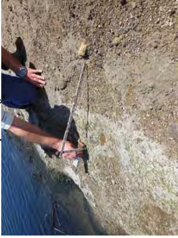
Photo 26: NP/SP - Erosion of ash material on common embankment south slope, looking west.
