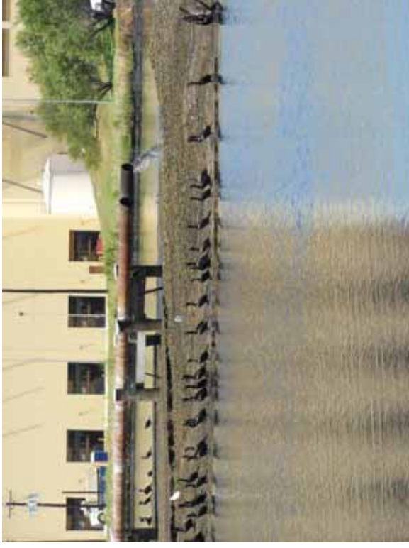
Photo 18: NP - Inlet piping, looking northwest. Piping includes one 8-inch diameter and two 12-inch-diameter pipes.
