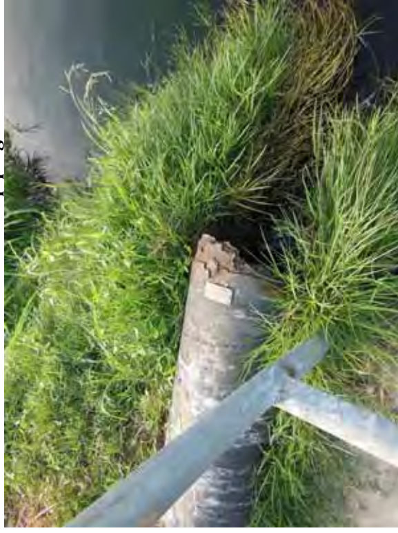
Photo 88: NP - 12-inch-diameter piping at outfall 103A.
